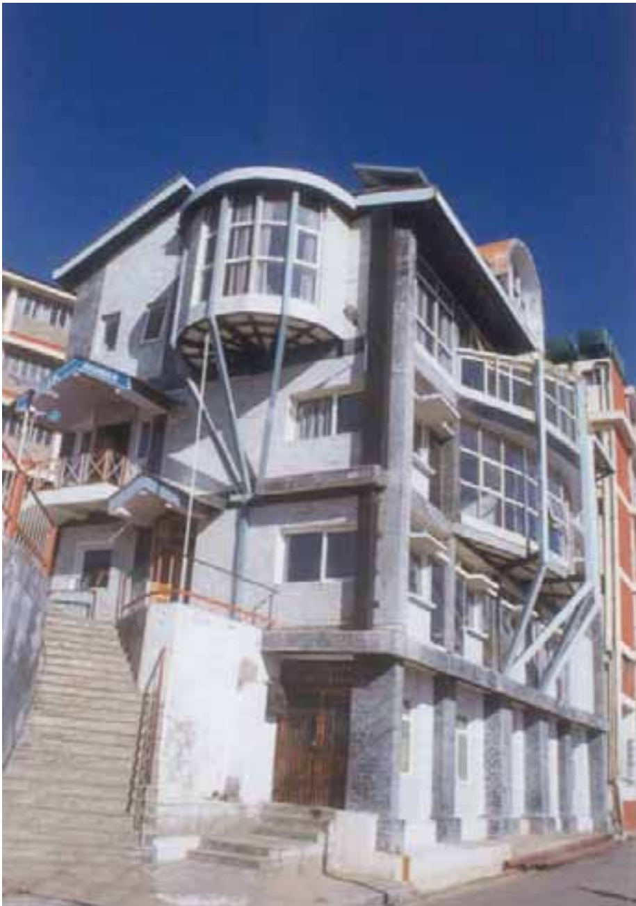
Himurja Office Building, Shimla
